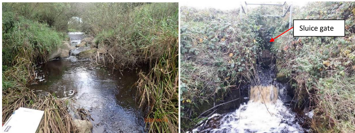
Plate 4 Reach of the Tarmon Stream downstream of Gabbet's Bridge (left): the bridge apron in the background is deemed an impassable obstacle for upstream migrating lampreys. The Tullamore Stream (right) drains the southern extent of the proposed development site and discharges to the River Galey. Note the fish passage problems associated with a sluice gate and a perched foundation.
